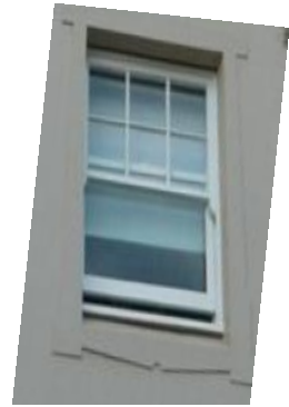
Timber frame & sill Timber awning sashes Double hung. Glazing bars top panels .
