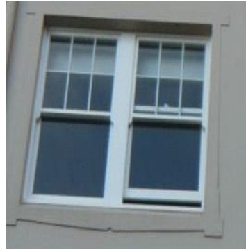
Timber frame & sill Timber awning sashes Double hung. Glazing bars top panels .
